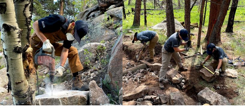
they focused most of their efforts on the heavily used and severely eroded sections of Cub Lake. The Corpsmembers also worked on the replacement of the trail's rock and wood steps which help to decrease water flow and thereby reduce erosion. The crew was also tasked with clearing drains and expanding the trail corridor for safe use for the recreational hikers and equestrians.
