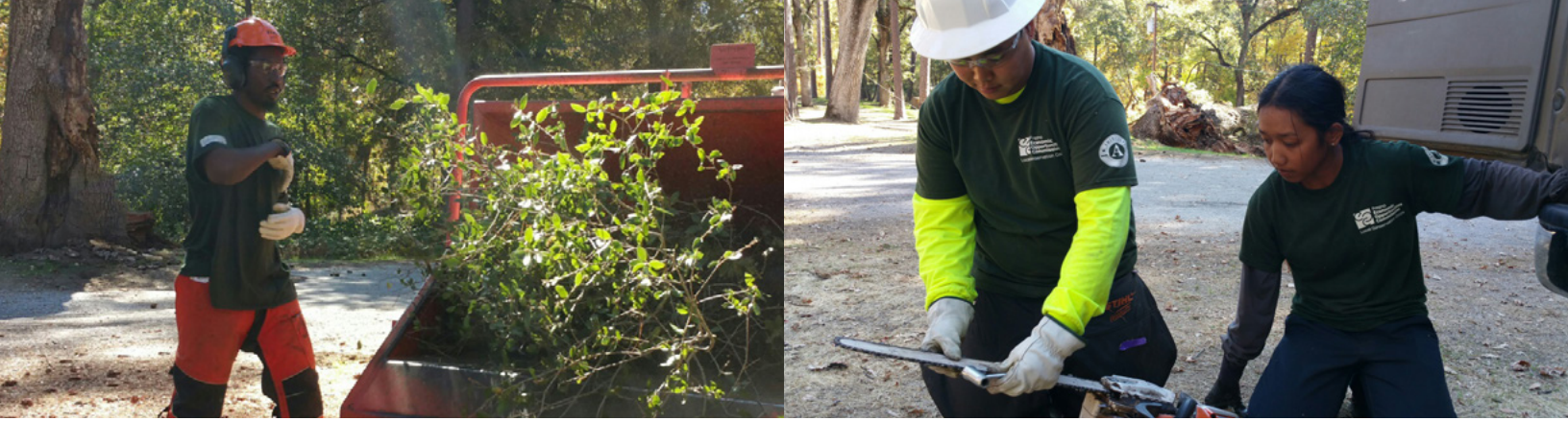
RTP Project: AmeriCorps members with Fresno Local Conservation Corps (CA) clearing brush along trails.
