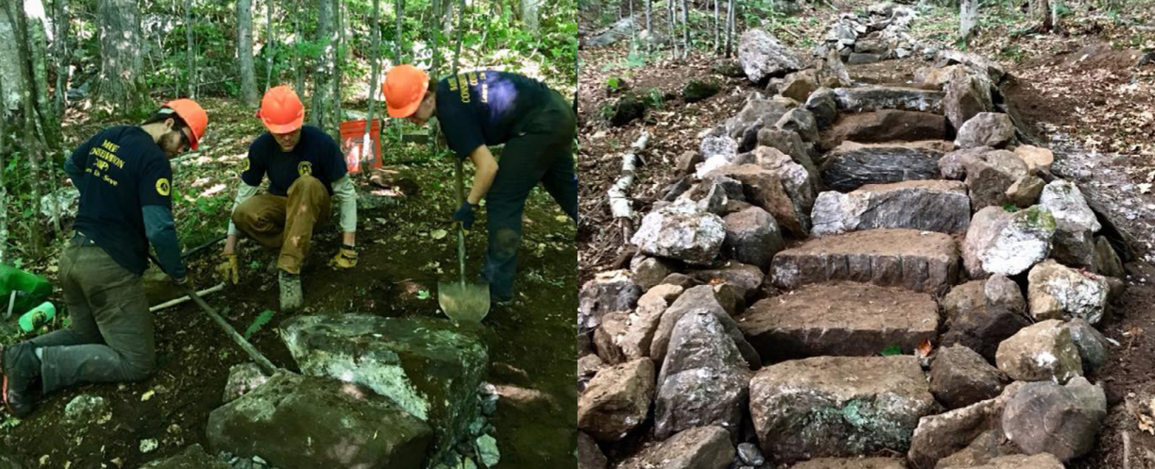
RTP Project: AmeriCorps members with Maine Conservation Corps; stone steps they installed at Grafton Notch State Park.
