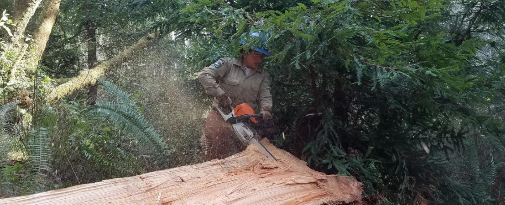
RTP Project: A Corpsmember with the California Conservation Corps serving on the Arcata Ridge Trail .
