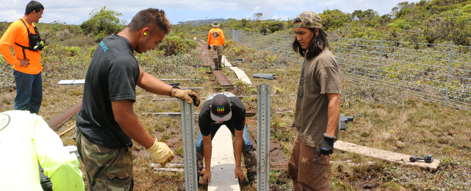
Installing new boardwalk sections on the Alaka'i Swamp Trail.
