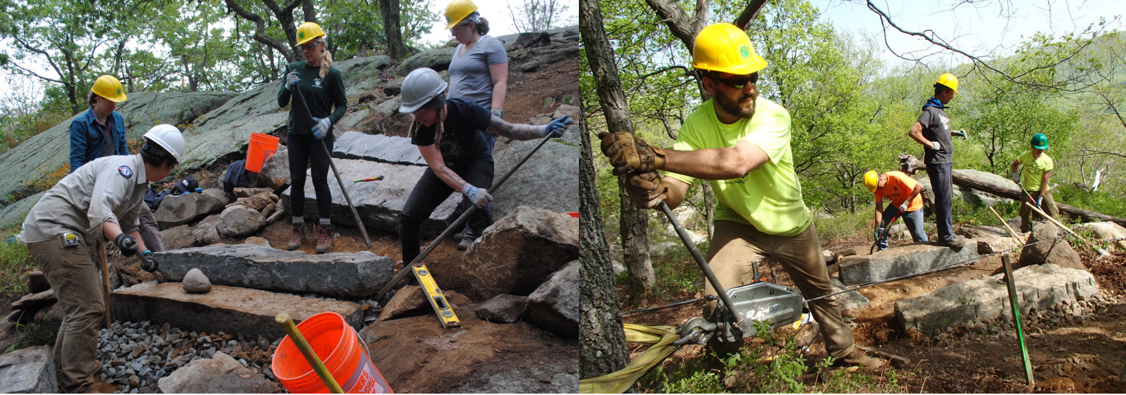
NYNJTC Conservation Corps Corpsmembers at work at Bear Mountain State Park.
