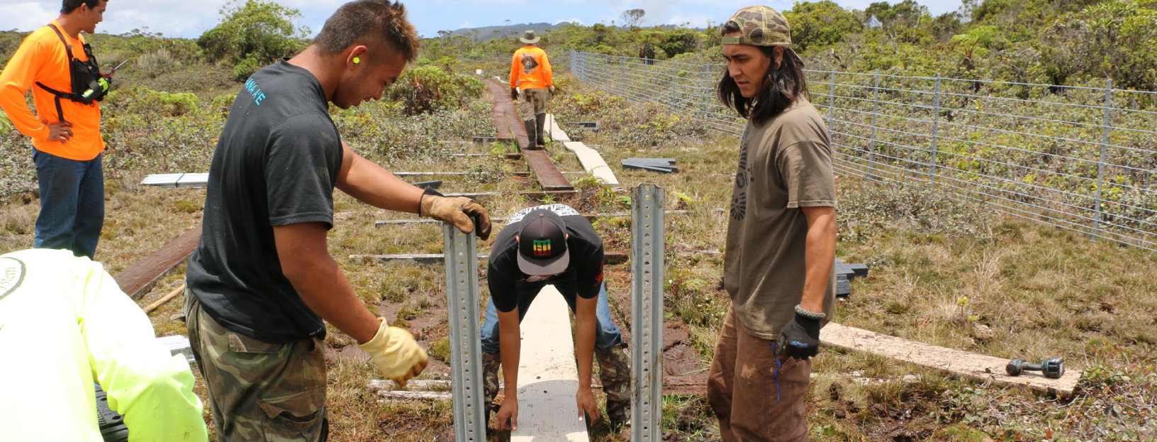
Kupu's boardwalk repair project on the Alakai Swamp Trail on Kauai (HI) is one of the Recreational Trails Program-supported projects featured in The Corps Network's new guide for trail managers interested in working with Corps.
