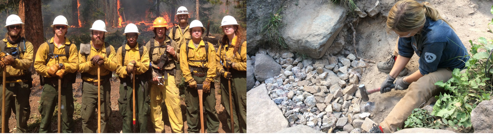
Left: Rocky Mountain Youth Corps-Colorado used The Corps Network's cooperative agreement to do fire fuel abatement work at Rocky Mountain National Park. Right: Larimer County Conservation Corps used the agreement to do trail work at the same park.
