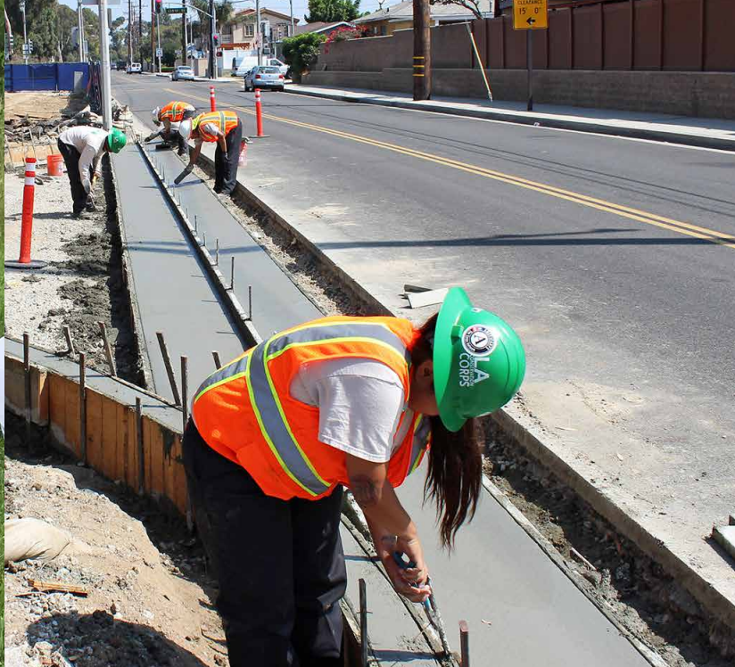
Left: Vermont Youth Conservation Corps Farm Corps members. Right: The Wiseburn Walking Path under construction. See below for a brief description of these 2018 Projects of the Year.
