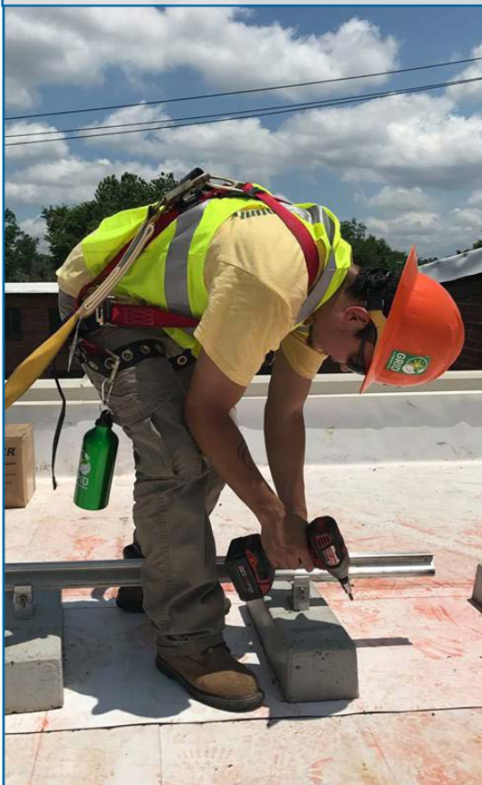
Montgomery County Conservation Corps, solar panel installation.
